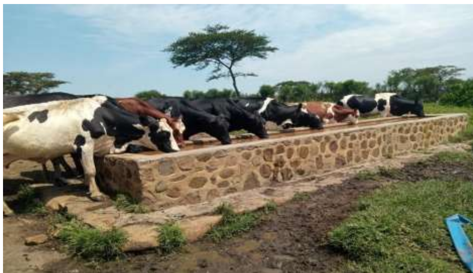
Figure 5-9: Status of existing water trough installed by the Project
