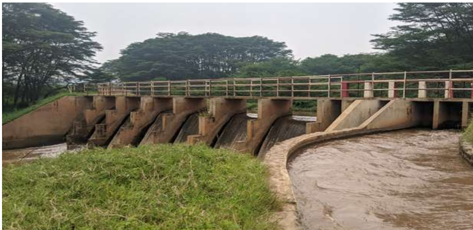
Figure 5-10: Muvumba Diversion weir, source of water for Muvumba P8
